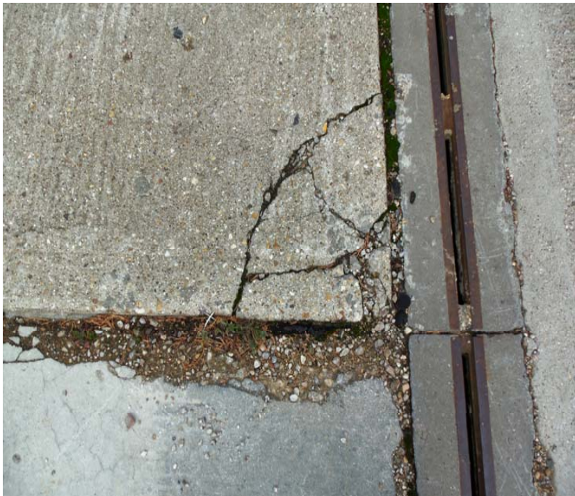
Corner cracking
