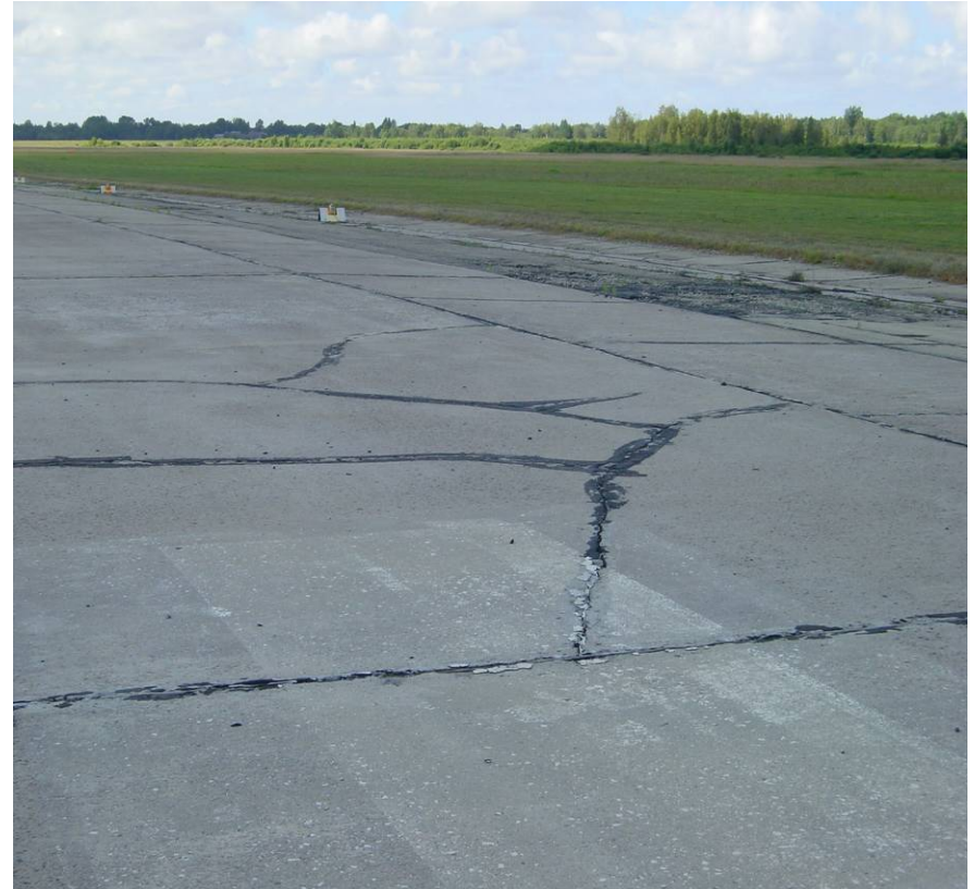
Bay cracking
