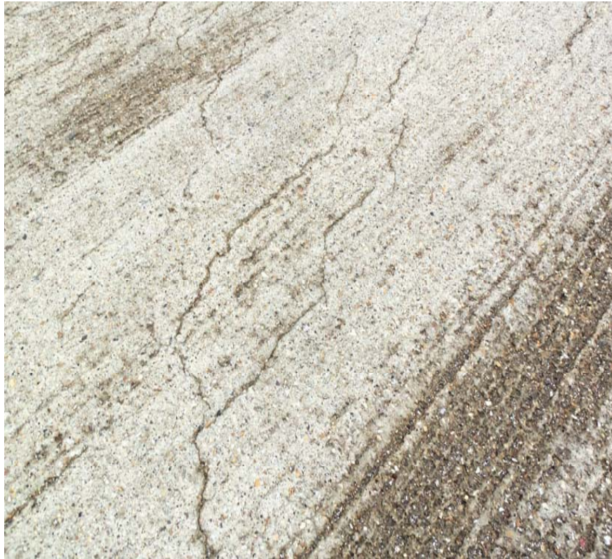
Shrinkage cracking
