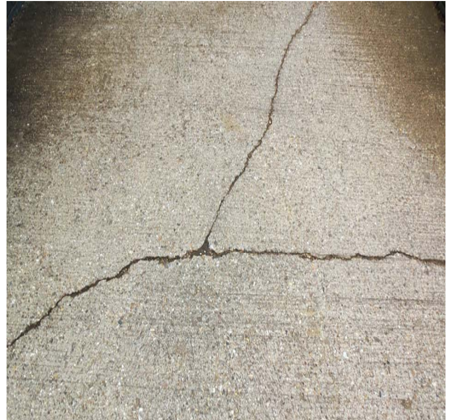
Settlement cracking
