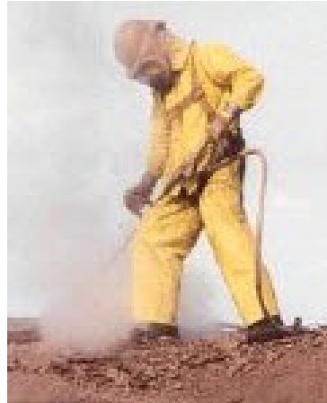
High pressure water blasting
