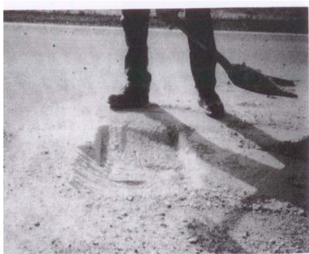
Figure 2. Recommended orientation of milled patch
