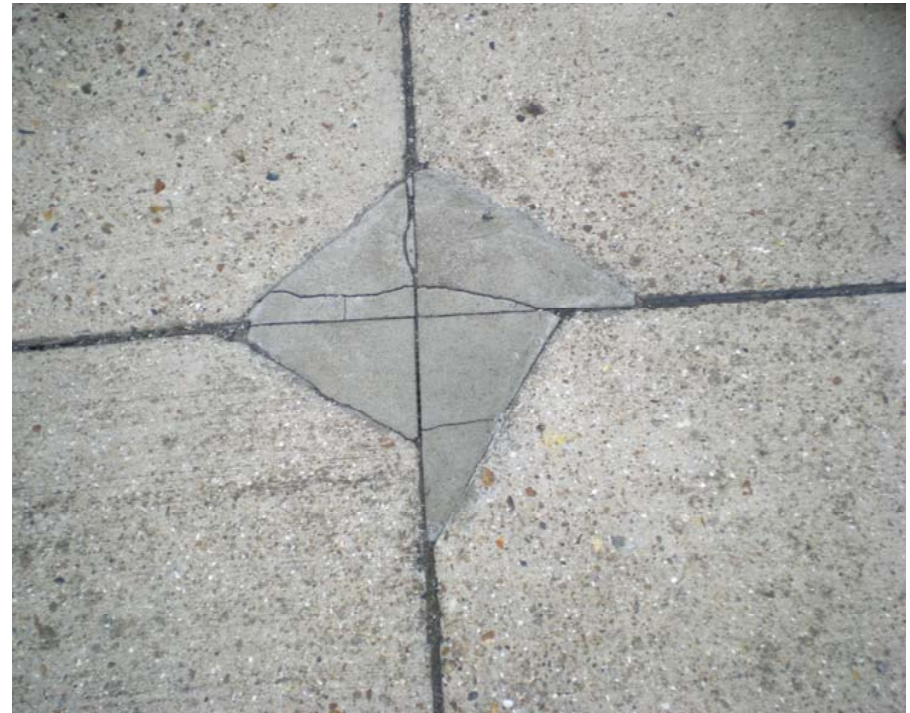
Poor repair
