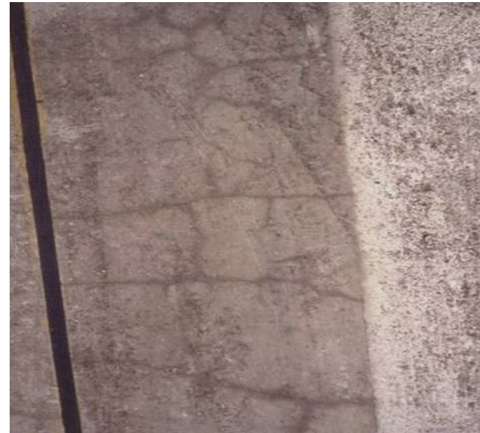
Shrinkage Cracks
