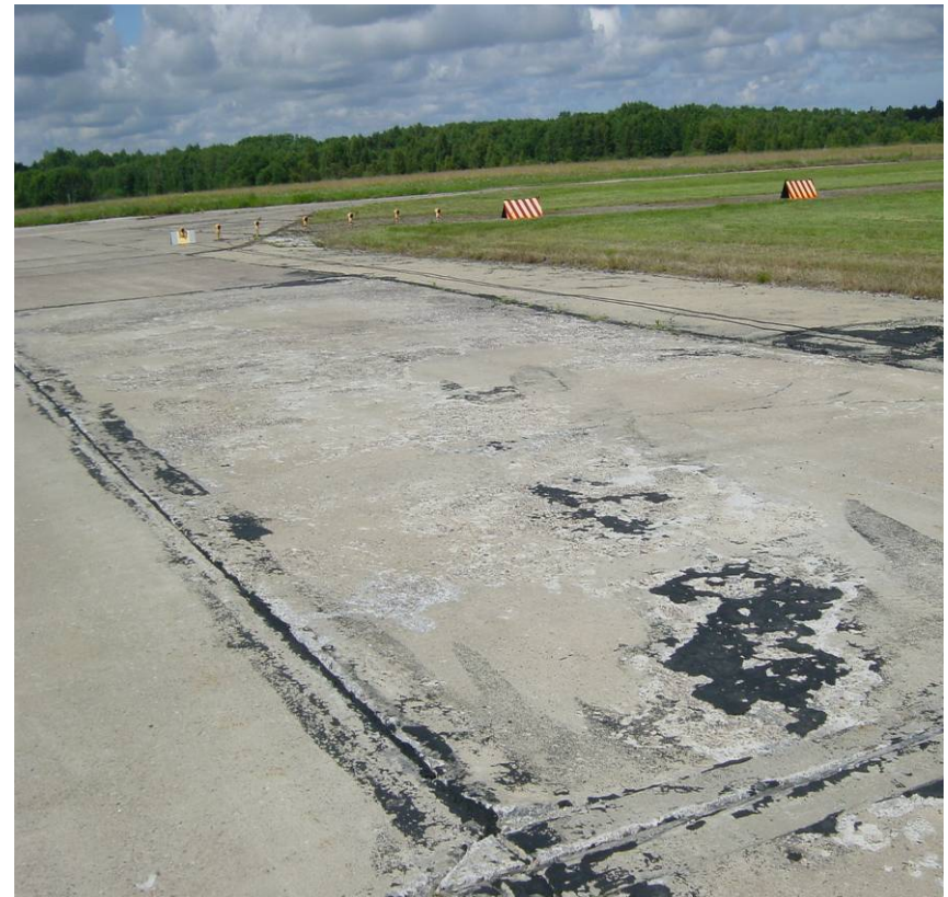
Poor repairs
