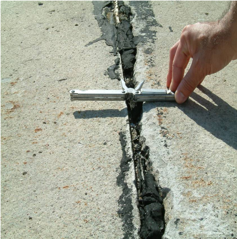
Defective joints
