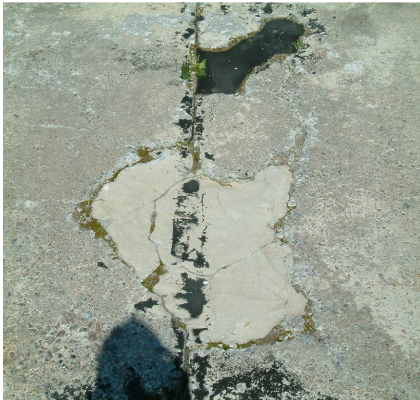
Poor repairs
